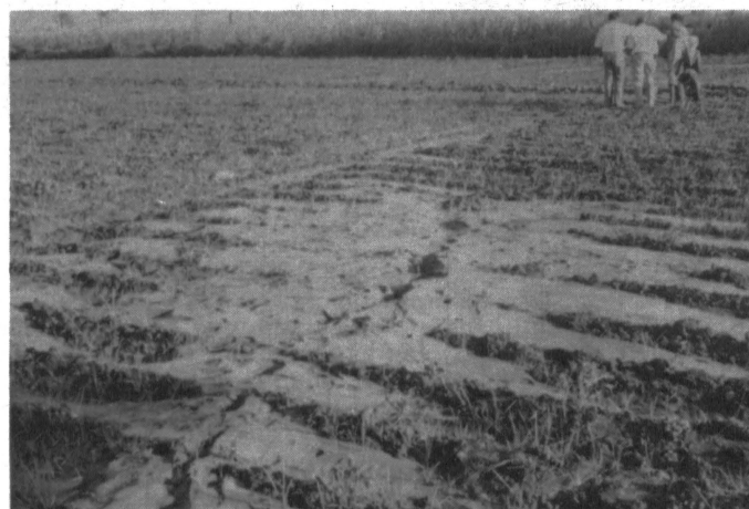
Fig. 6. Ground fissure and sediment eruption.
