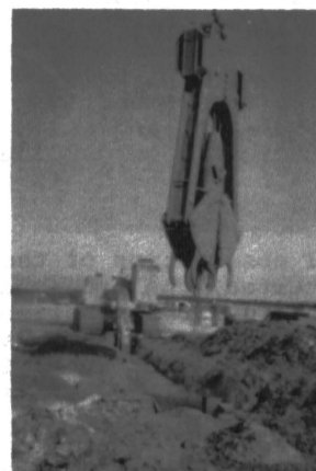
Figure 3. Installation of slurry trench and sheet-piles.
