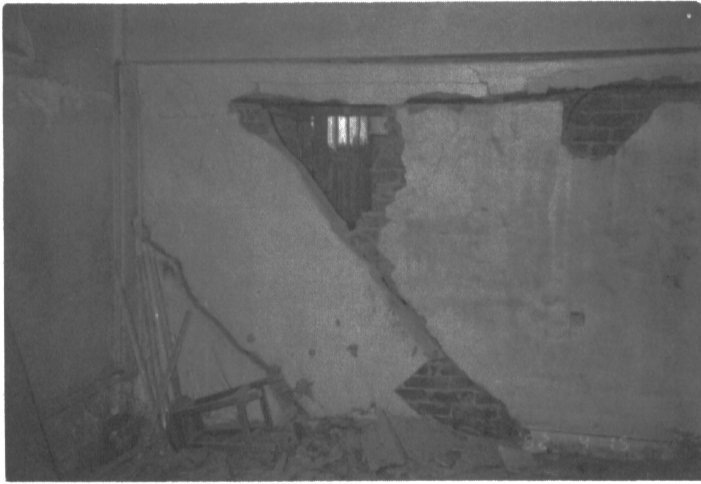
Photo 6 Example of Severe Cracks in the Internal Walls at the Basement of Main Building.
