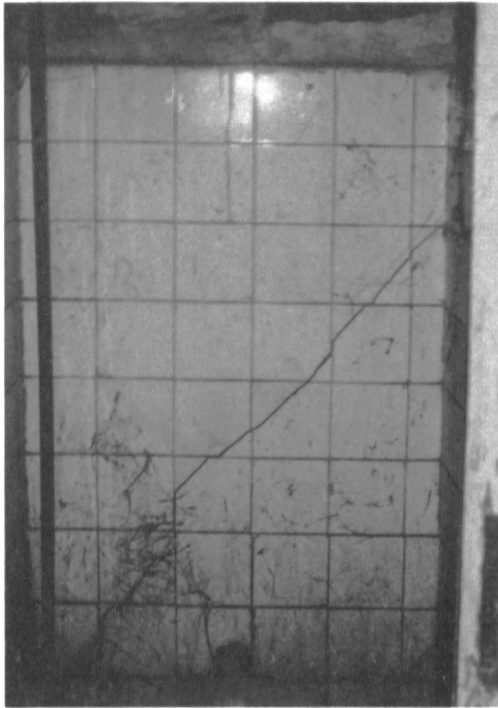
Photo 2 Example of Diagonal Cracks Inside Water Closets.
