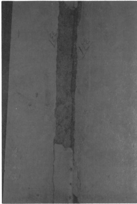
Photo 10 Example of Separation at the Location of Expansion Joints.
