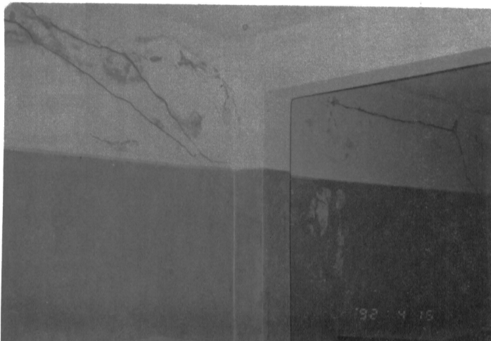
Photo 7 Example of Cracks in Beams at the Basement of Main Building.
