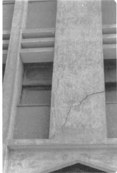
Photo 5 Example of Cracks in External Walls of Main Building.
