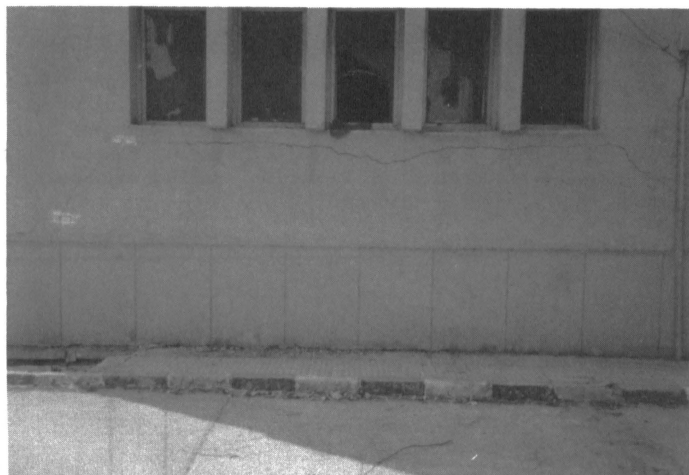
Fig. 2. Horizontal Crack in the Facade
