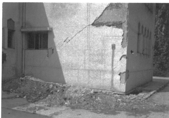
Fig. 3. Inclined Cracks in Walls
