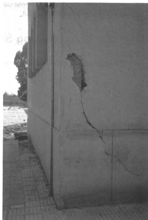
Fig. 4. Cracks in Columns and Walls
