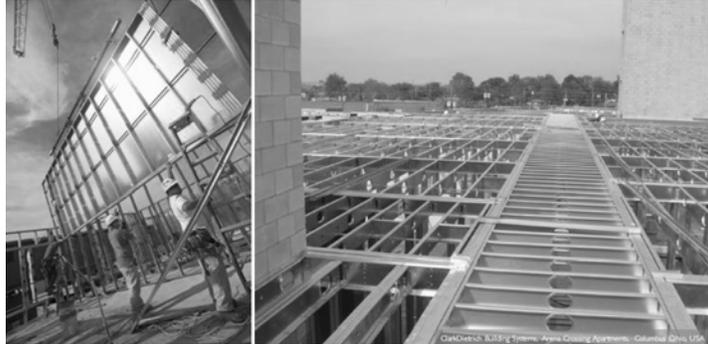
Figure 1: Cold-Formed Steel Framing
