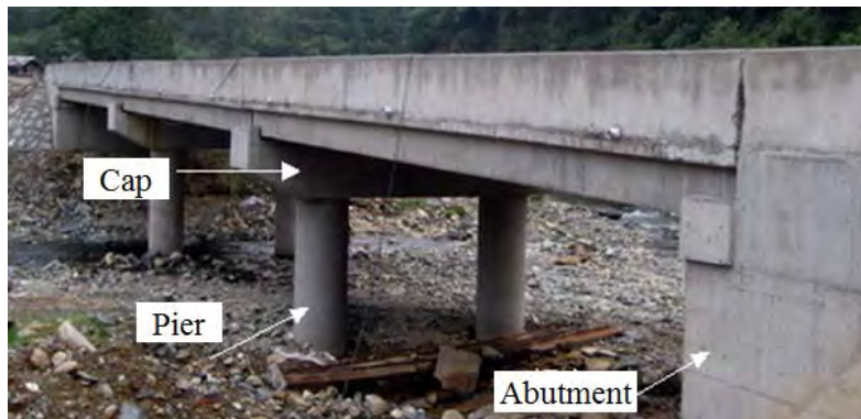
Fig. 2.1 Three-span prestressed concrete bridge.
