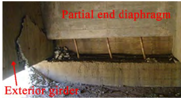
Fig. 3.15 San Nicholas bridge with partial diaphragms.
