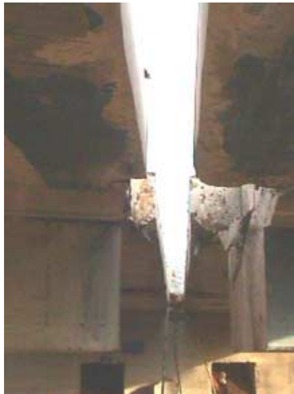
Figure 3.3. The bridge deck and a cap beam after cutting and removing concrete.
