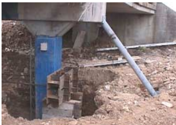
Figure 3.18. Diagonal bracing of the failed column.
