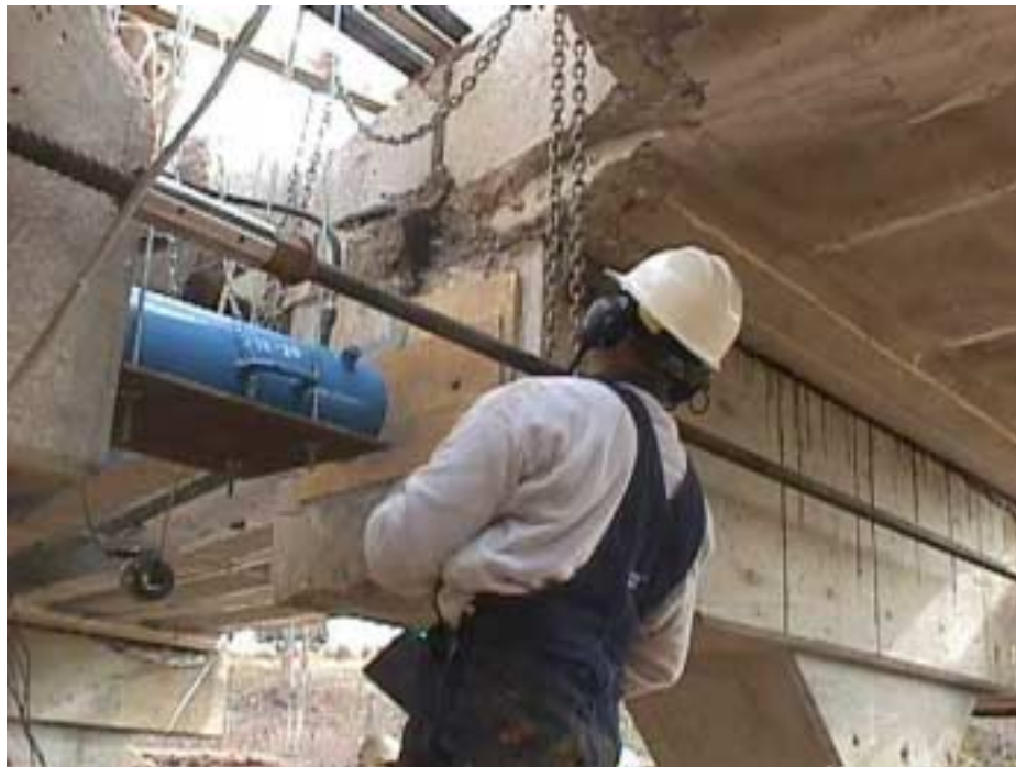
Figure 3.9. Placing the middle jack.
