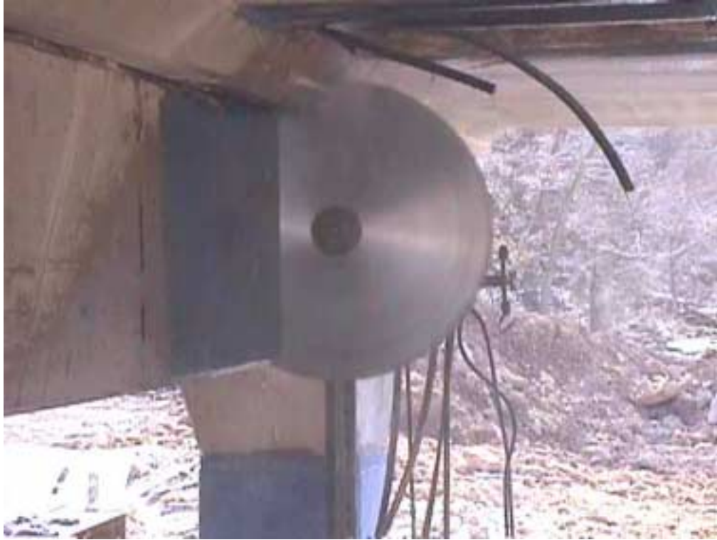
Figure 3.2. Cutting the cap beam.
