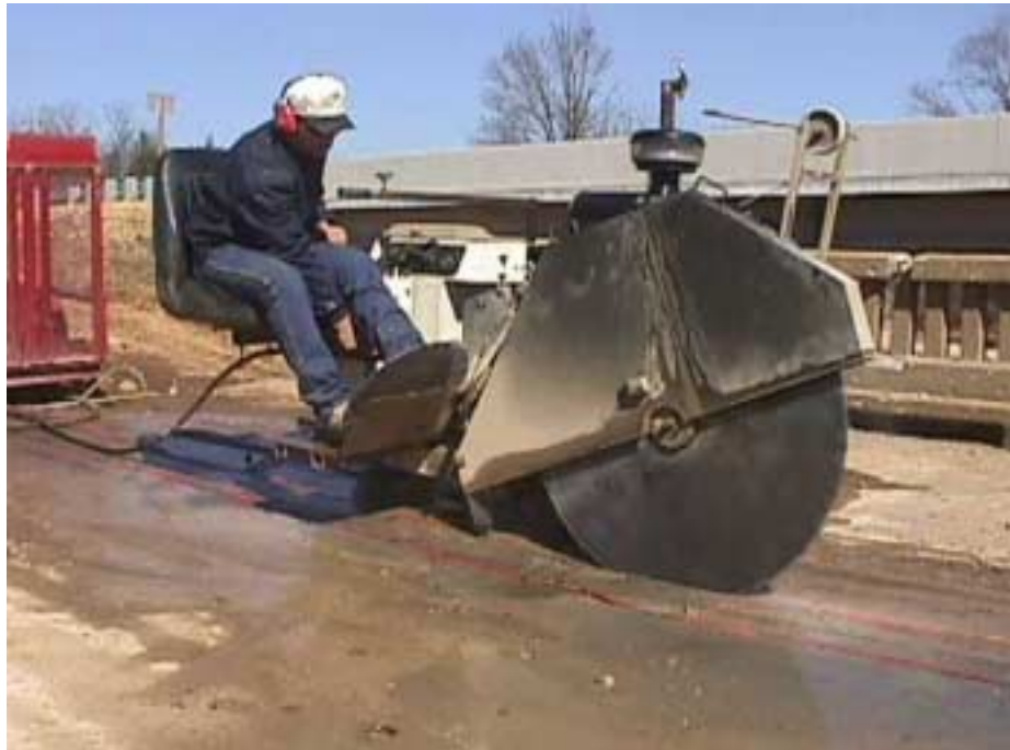
Figure 3.1. Cutting the bridge deck.
