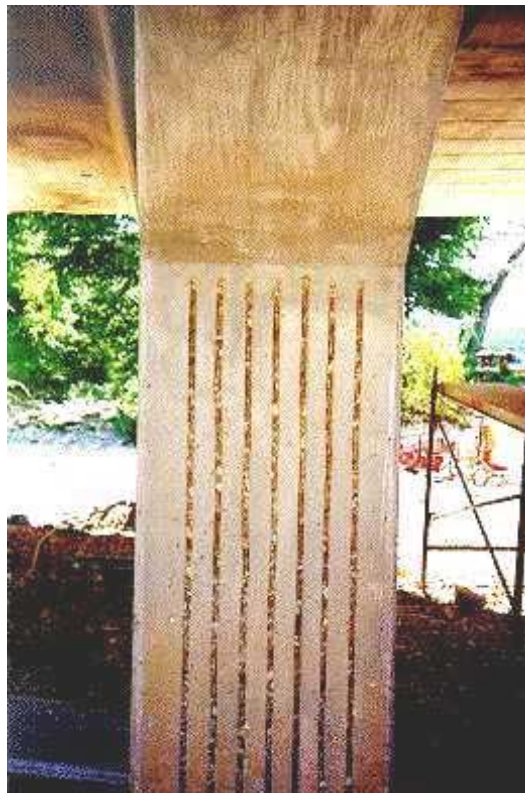
Figure 2.8. Grooves on the side of column B2P2.
