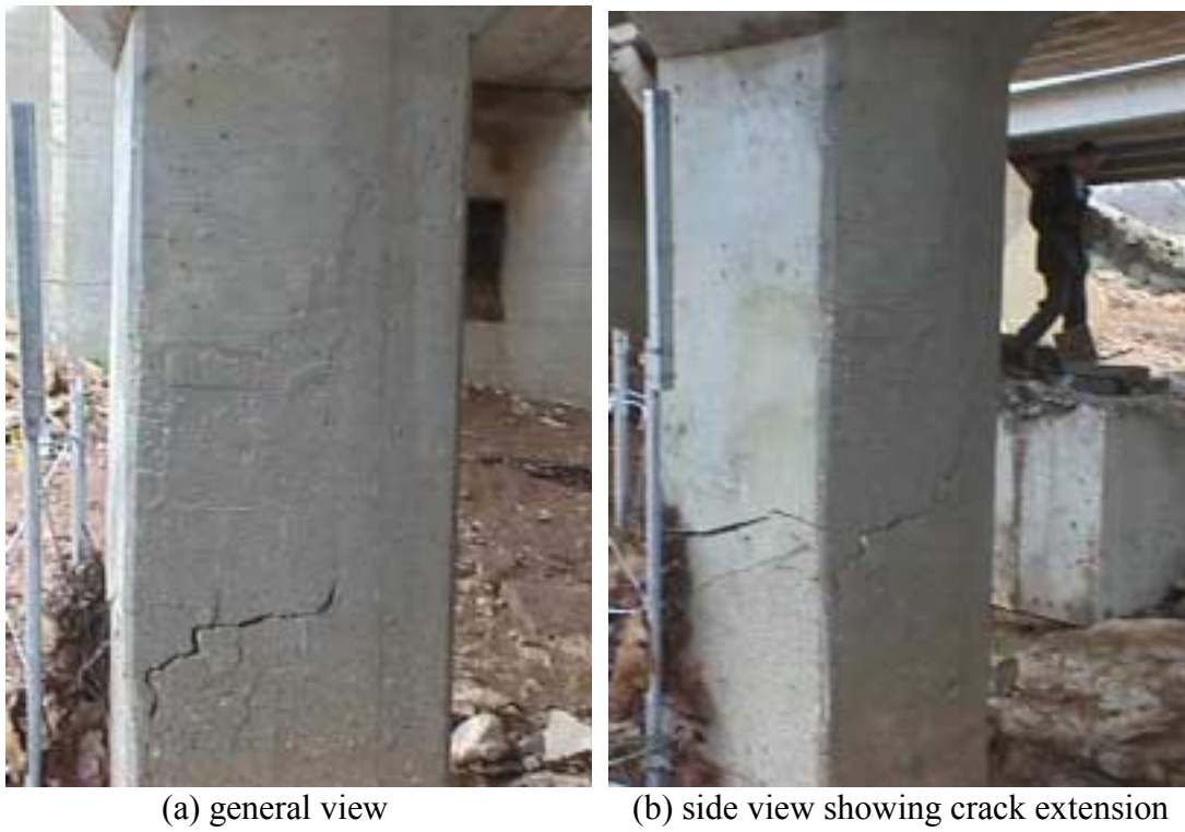
Figure 4.7. Crack on Column B2P1.
