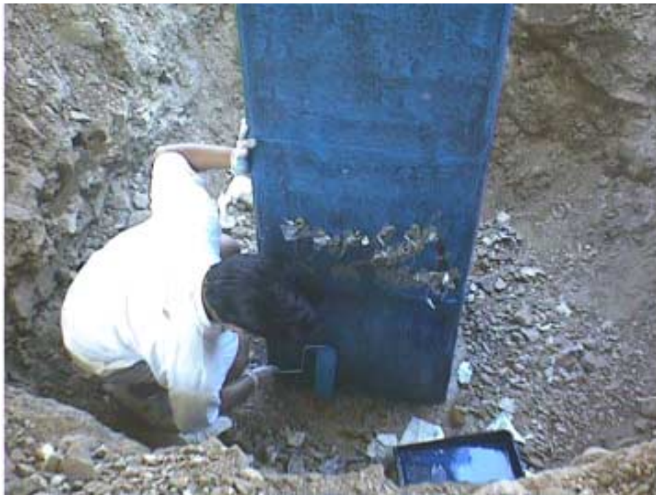
Figure 2.11. Applying the bottom lift of the jacket.
