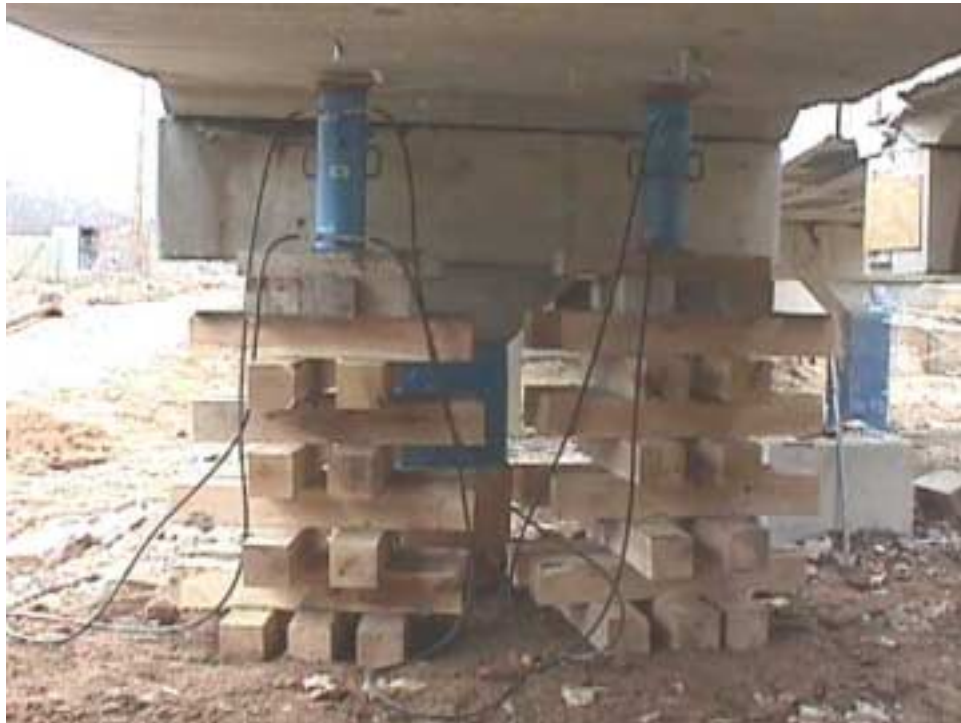
Figure 3.12. Set up for jacking the decks.
