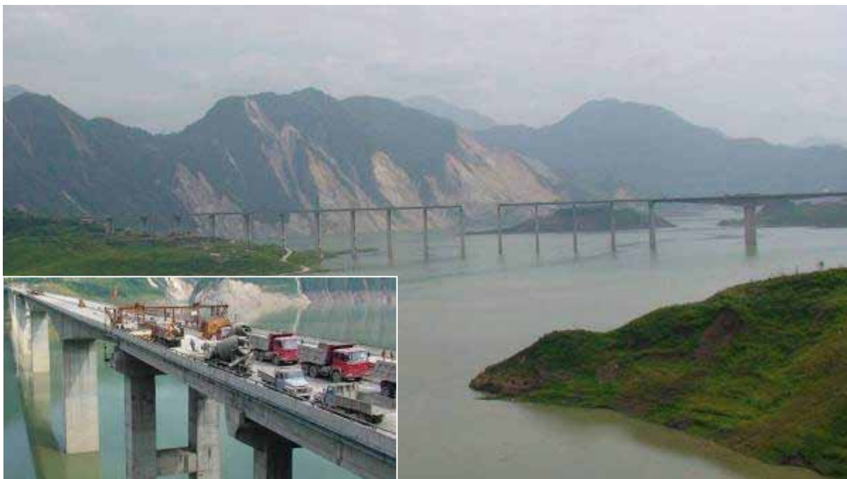
Figure 54. Photo. Overview of Miaozihiping Bridge.
