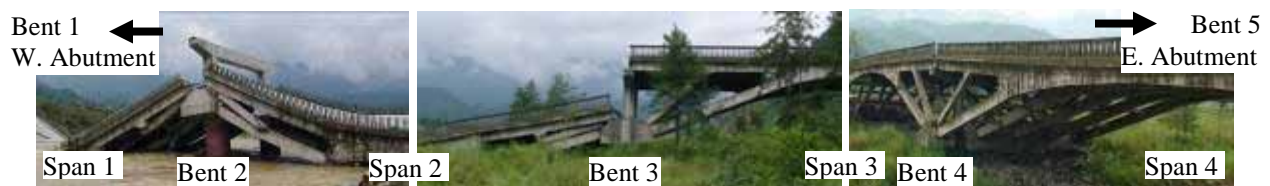
Figure 17. Photo. Overall View of the Remaining Arches.
