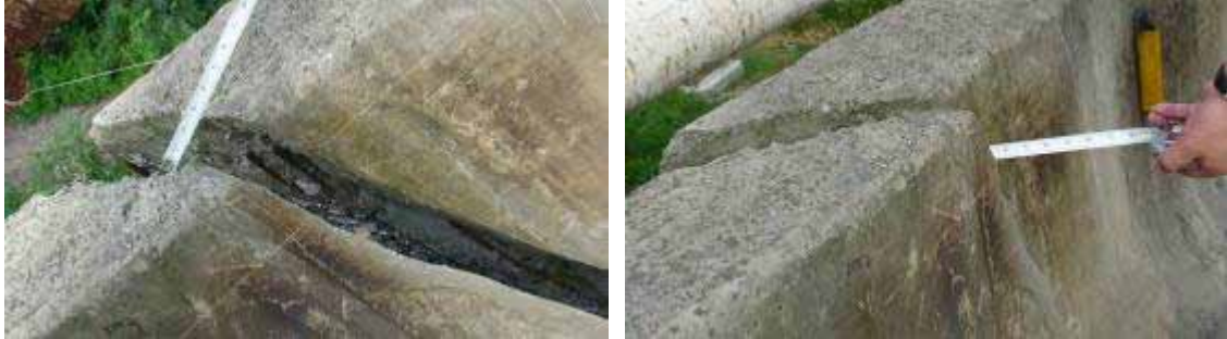
Figure 32. Photo. Measurement of Expansion Joint Offset.
