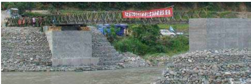
Figure 50. Photo. Bailey Bridge in Place.
