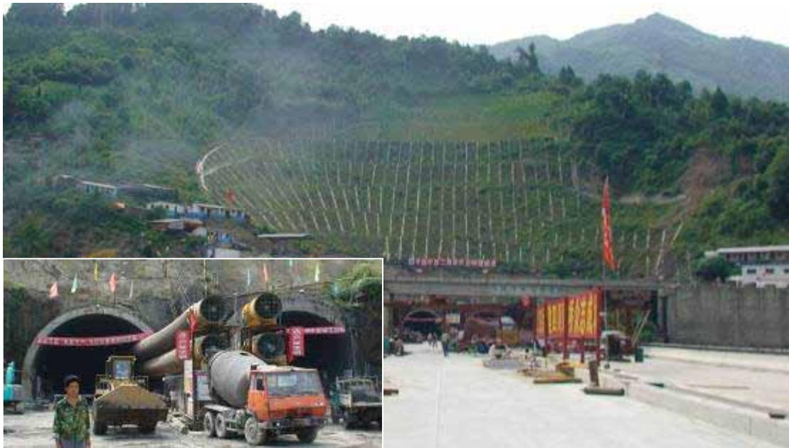
Figure 53. Photo. Miaozihiping Tunnel.
