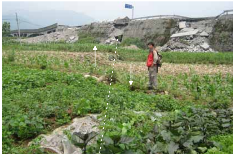
Figure 7. Photo. Surface Rupture Near Xiaoyudong Bridge.
