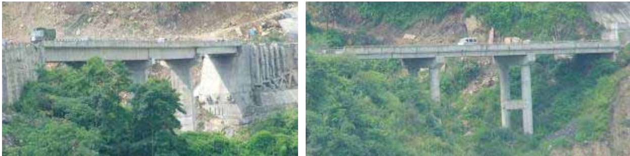
Figure 60. Photo. Bridges in the Vicinity of Miaozhiping Bridge.
