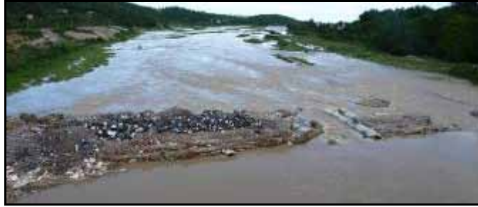
Figure 29. Photo. Temporary Roadway over the River.
