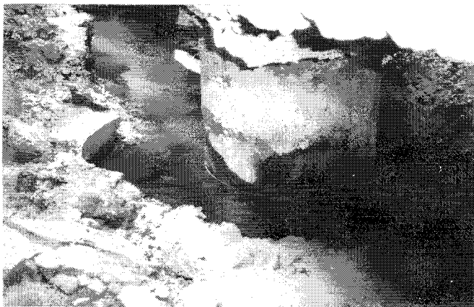
Fig. 8 Undamaged pile supporting a crane rail in ground which moved more than 1.0m.
