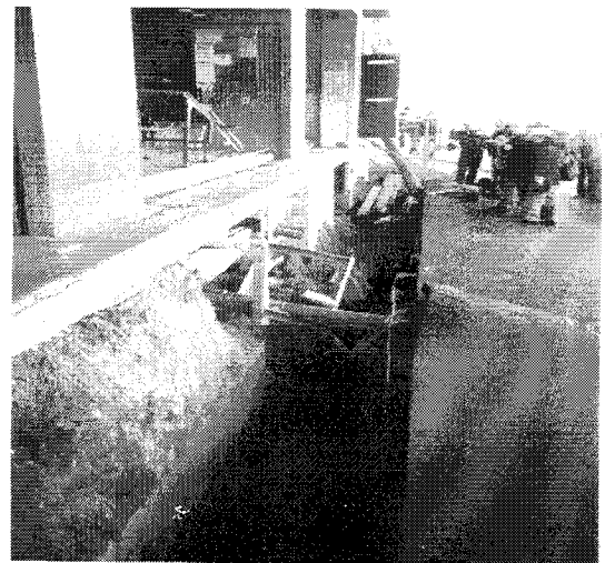
Fig. 6. Large ground displacements around the ferry building on Port Island after the Kobe earthquake, 1995.
