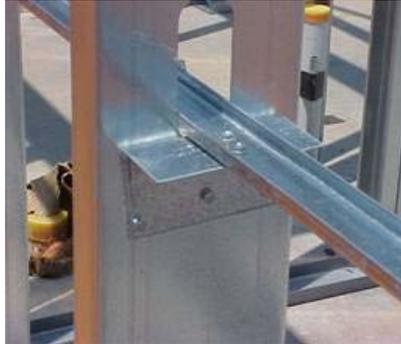
Figure 1: Generic connector used with bridging
