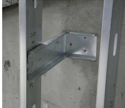
Figure 2: Field-fabricated curtain-wall connector
