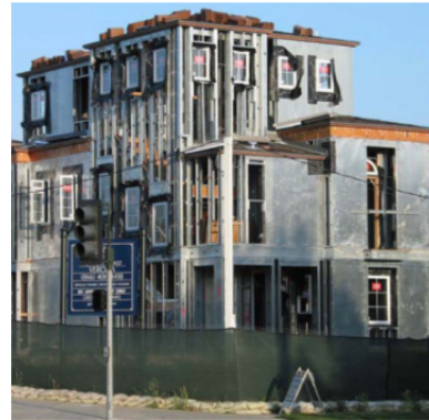
Figure 2: CFS shear walls using sheet steel sheathing (Courtesy of Simpson Strong Tie)
