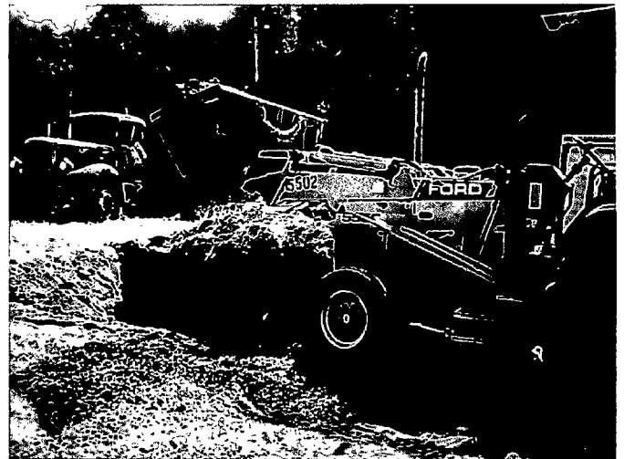
Fig. 2 – Crushed Rock Dumped into Test Trench
