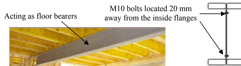
Figure 2: Back to back built-up LSBs (LST, 2005)
