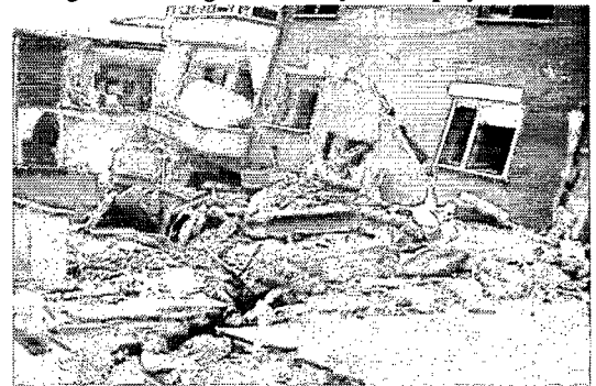
Fig. 8. Damage caused by soil liquefaction.
