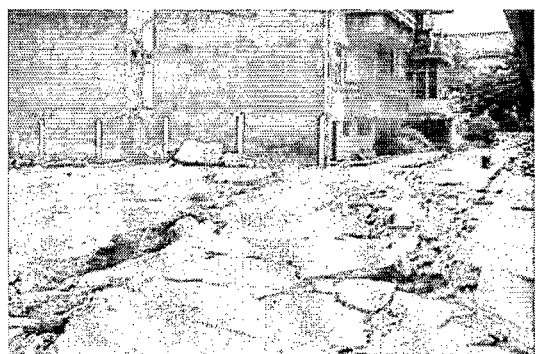
Fig. 9. Damage caused by large ground fissure
