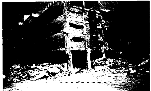
Fig. 4 Hotel collapse at "Valimitika", 15 June 1995.
