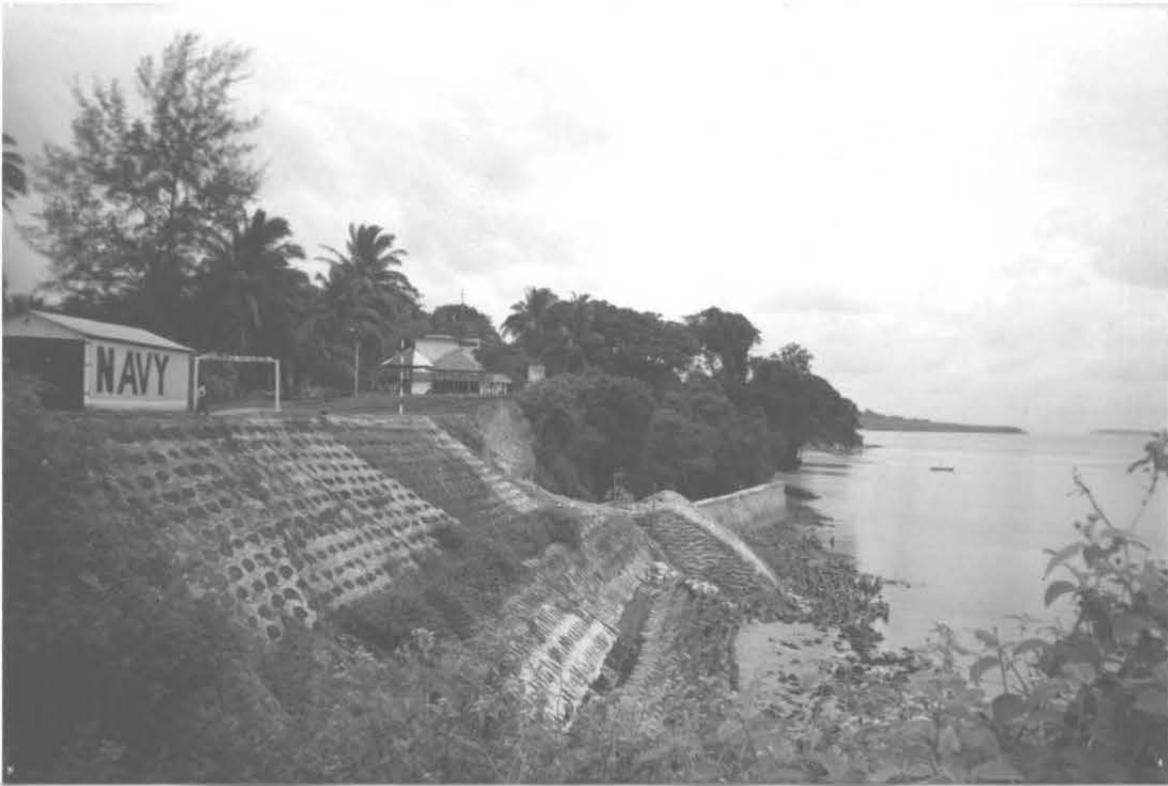
Fig. 4 Completed Gravity Sea Wall With Revetment and PCC Wall Partly Constructed
