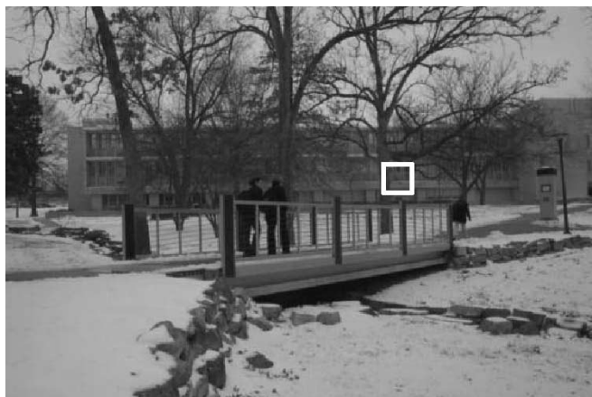
Fig. 1. Smart Composite Bridge at the UMR. The location of the dedicated Web camera is indicated on the building in the background.
