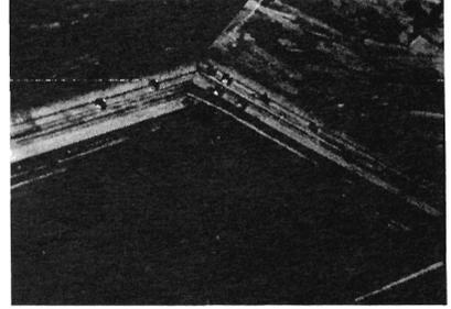
Fig. 8(c) Connections details at the top of the King Post
