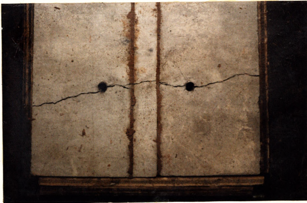
Figure D-14: 1/16 in. Clay Filled, Two-Joint Concrete Model Test: Test C-31, S=3 7/8 in., A Success
