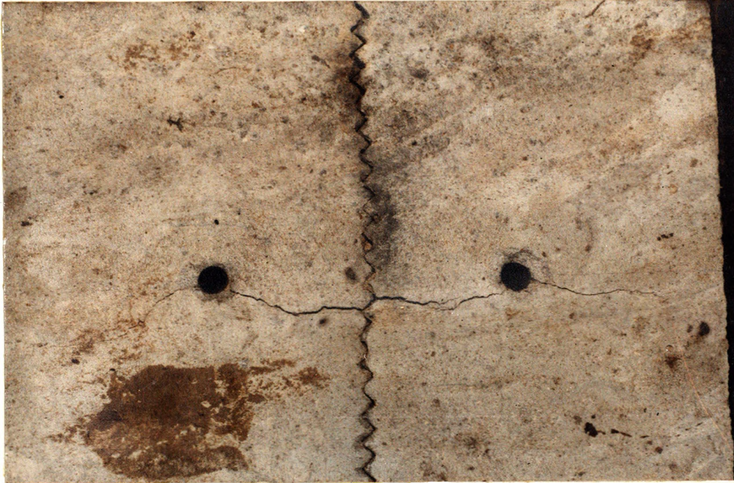
Figure D-19: Grooved Discontinuity Concrete Model Test: Test C-43, S=4 \frac{7}{8} in., A Failure. Split Extended to the Grooves' Bottom
