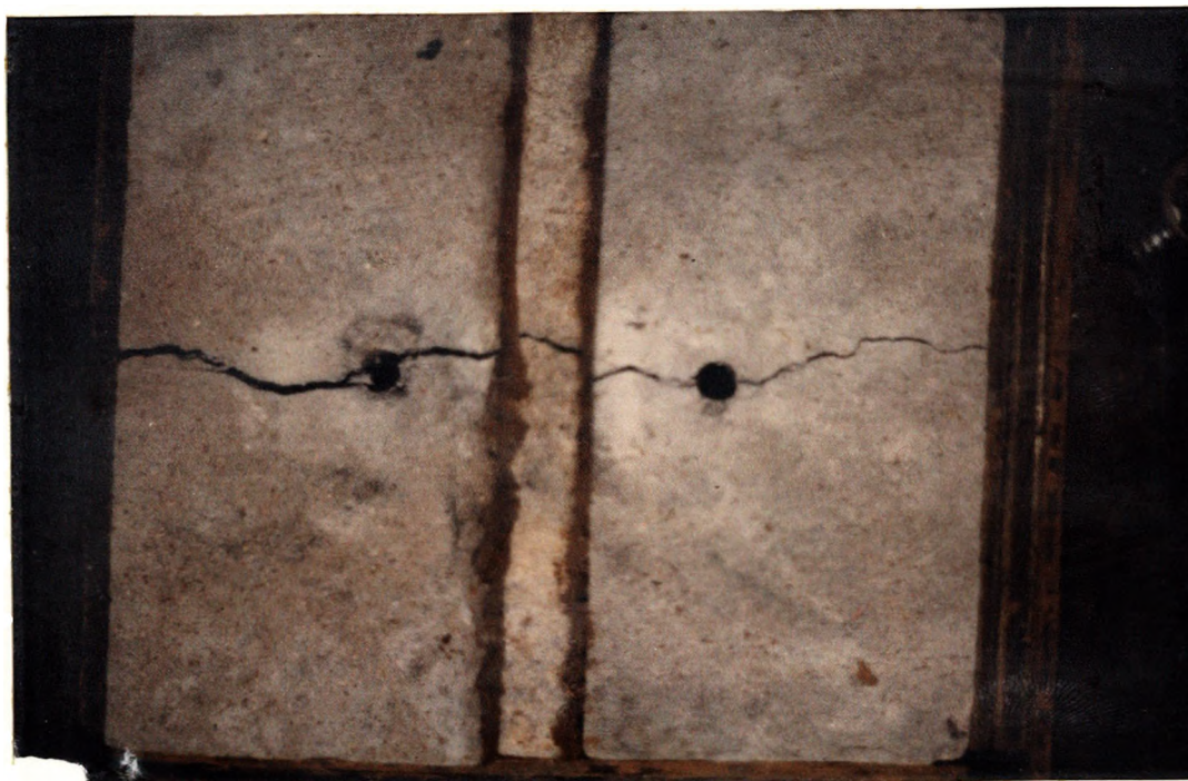
Figure D-18: 1/4 in. Clay Filled, Two-Joint Concrete Model Test: Test C-41, S=3 5/8 in., A Success
