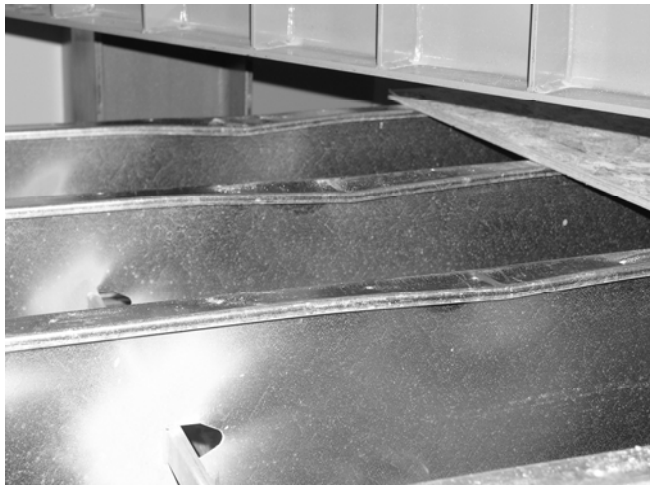
Figure 11 Photograph of failure in C-section Floor
