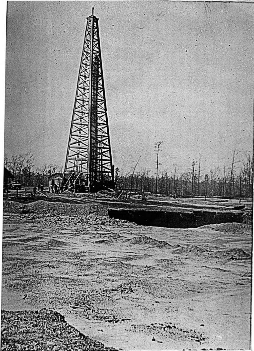
The crater of the Louisiana Oil Refining Corporation's Gleason No. A-1, in sec. 19, T.22N., R.9W., showing the derrick of the relief well, Gleason No. A-2. Gleason No. 1, the discovery well, was drilled too deep and abandoned.
