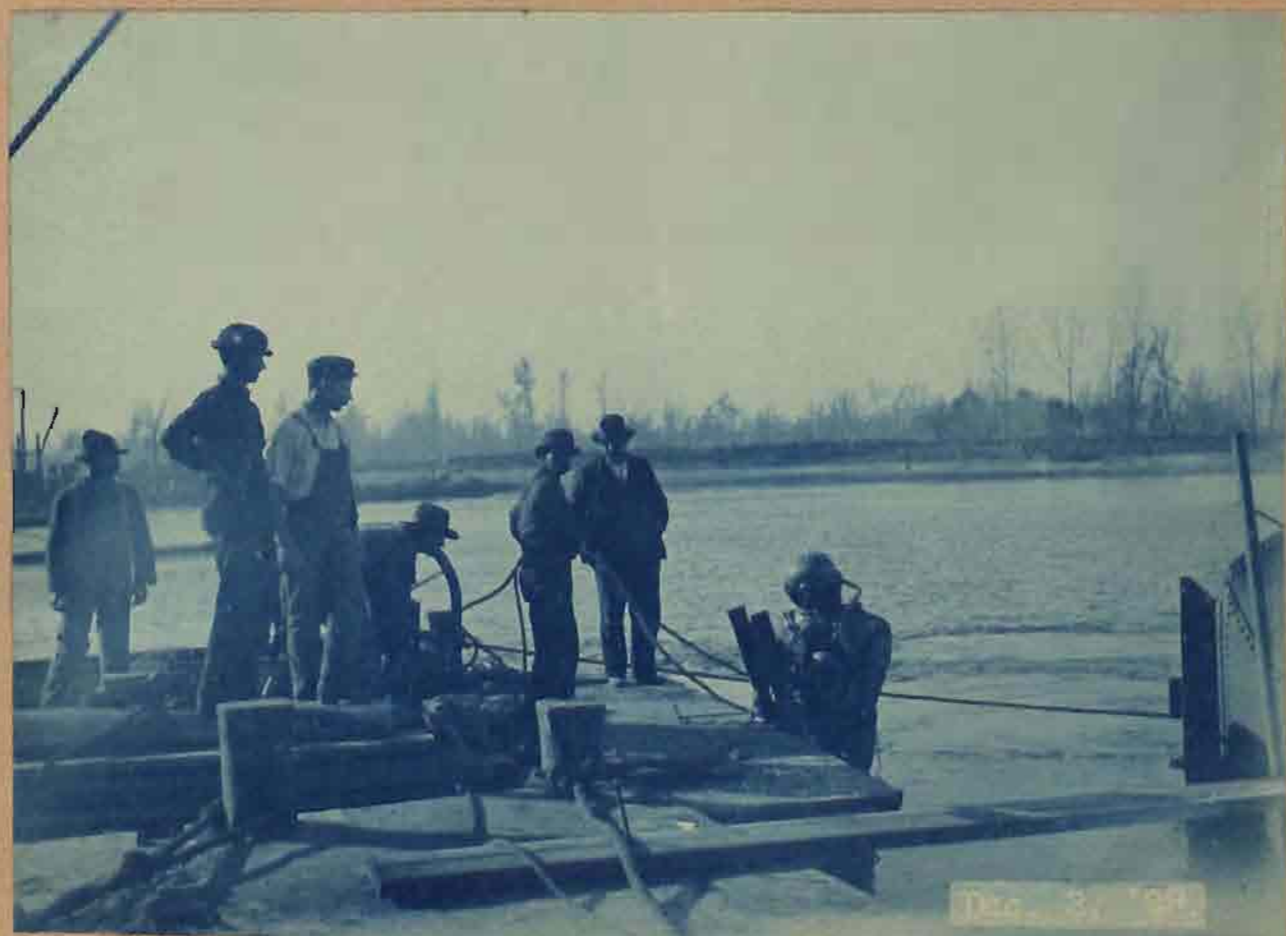
Diver going under water to unbolt clay-hoist off of shaft, which is in danger of being swept away by high water.
