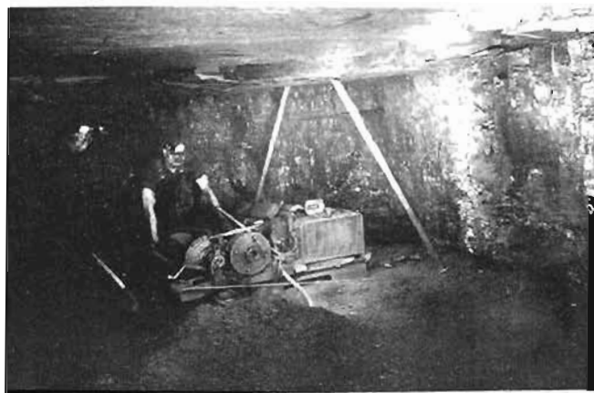
The seam is undercut in the usual manner.
