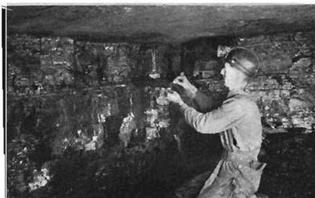
The Cardox tube is inserted in the drill hole with the discharge end at the back of the hole. The electrical terminals in the head of the tube are connected to a regular shot firing cable.
