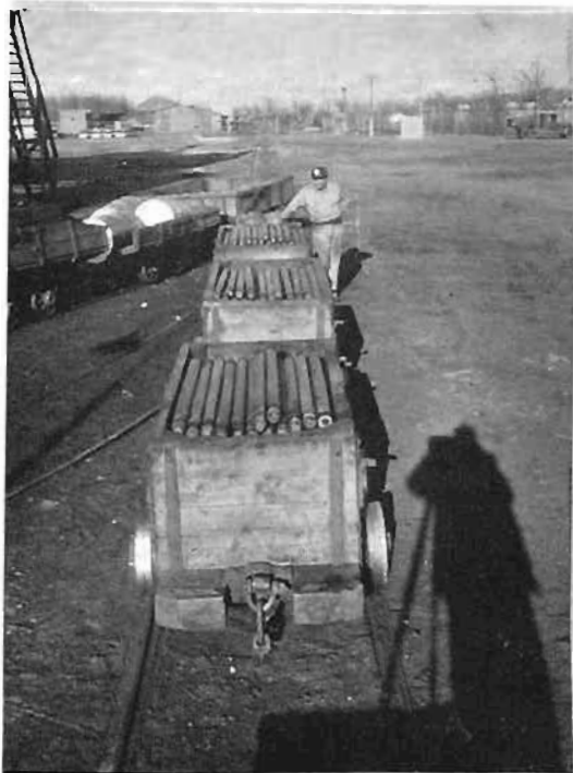
Charged Cardox tubes are sent into the mine in trucks constructed for that purpose.
