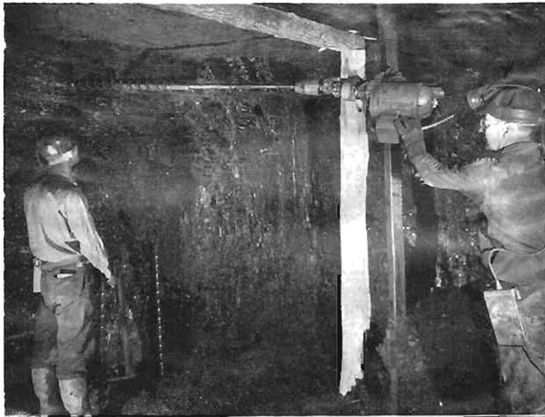
Drilling the hole for a Cardox tube.
