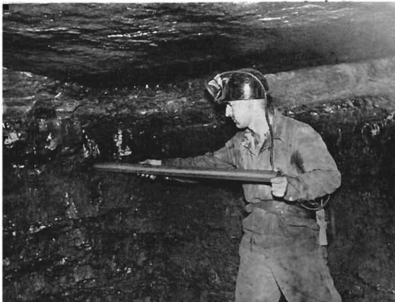
Inserting a Cardox tube in the drill hole. Figure 6
