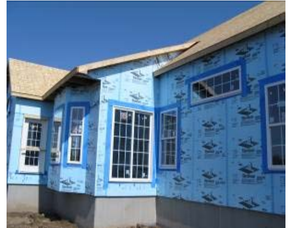
Image 2.1: Home covered with 2 inches of rigid foam in New York
