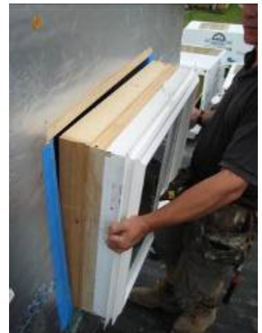
Image 2.4: Extension Jambs attached directly to a window
