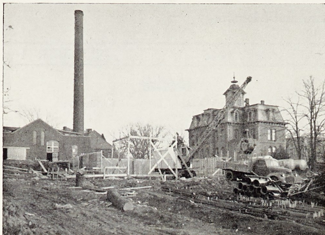
(Construction work on new power plant on January 4, 1946)
