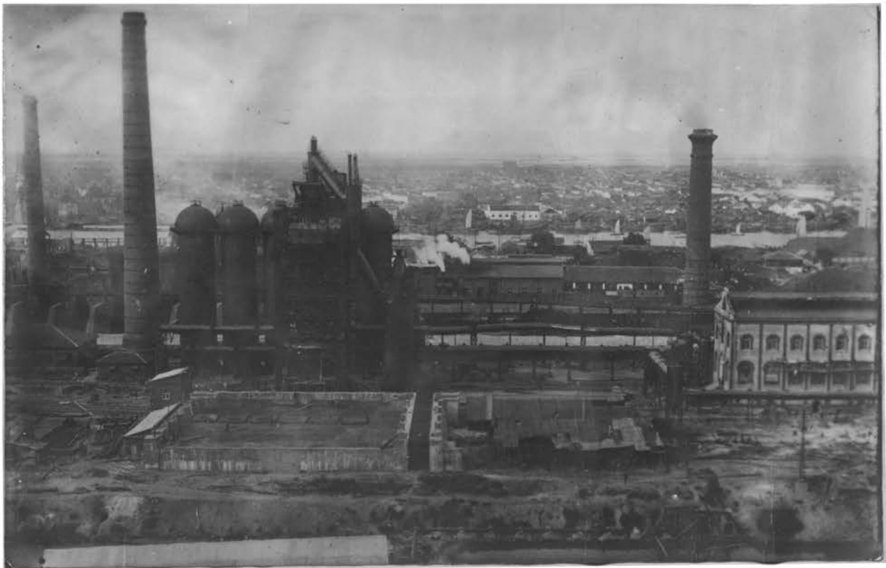
5-Another General View of Plant, New Furnace in Background to left; Old Furnace just back of it, and Hankow in distance (across the Hsi Kiang).
