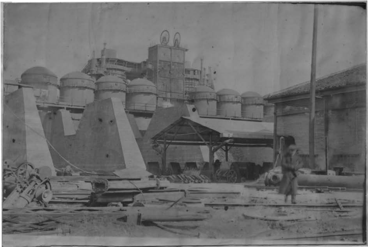
2-Blast Furnaces which are now in Operation--One- storage compartments just in front of Furnaces.
