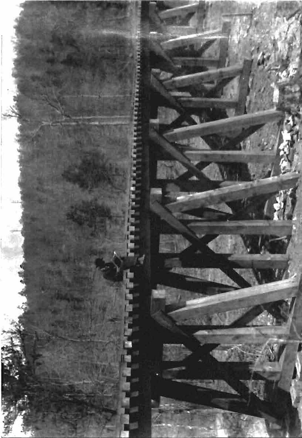
Illustration No.1 Framed Bent of Square Timbers.
