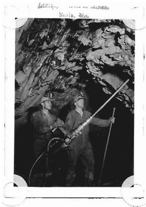
Drilling Side-Swipe Holes
