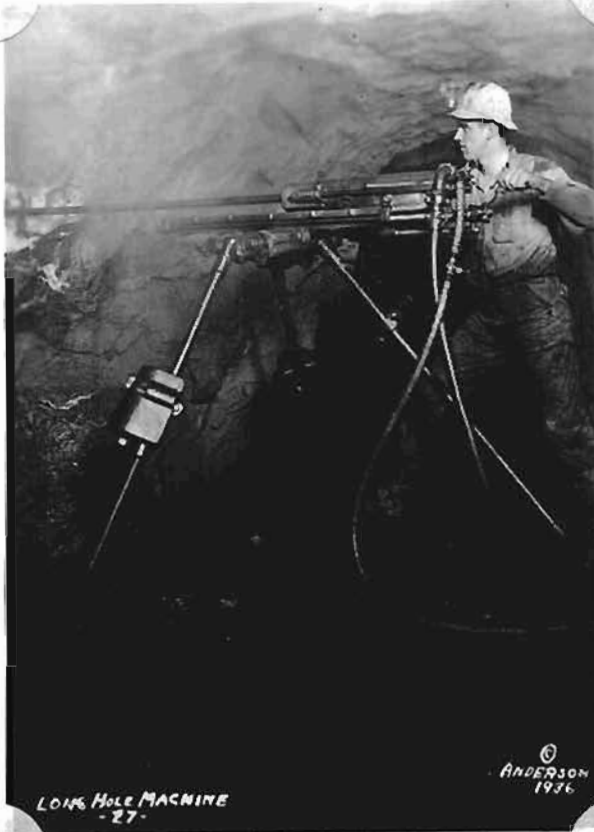
DRILLING LONG HOLES Two Types of Mounting for the Long-Hole Leyner Drills
