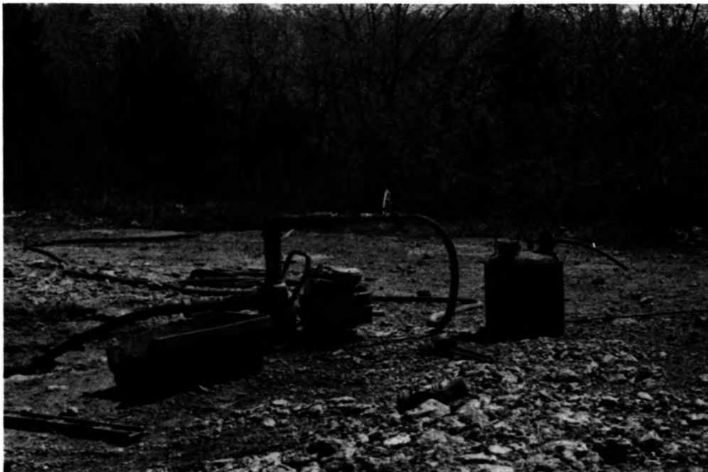
Figure 5. Gasoline-Powered Pumps Used For Water Removal
