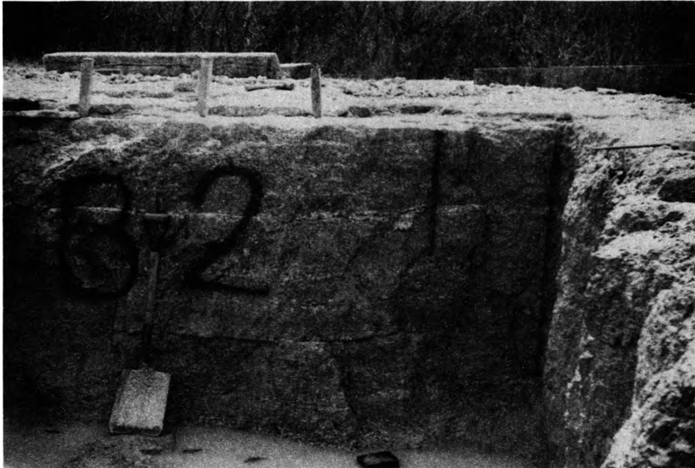
Figure E-13. Bench for Test B-2 Before Blasting
