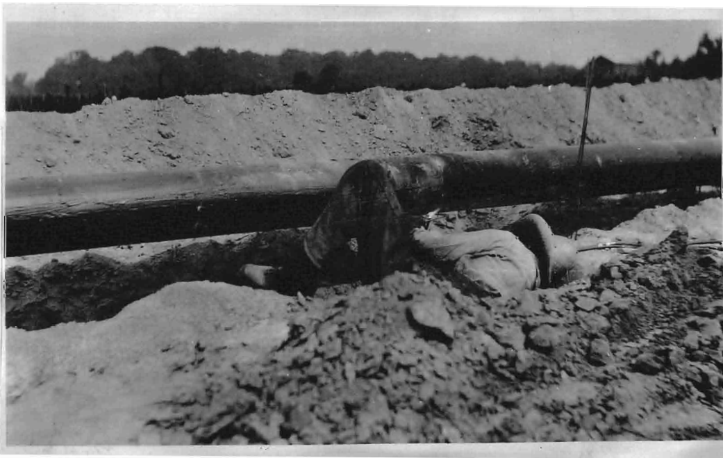
Making an Overhead Weld on a 10" Line
