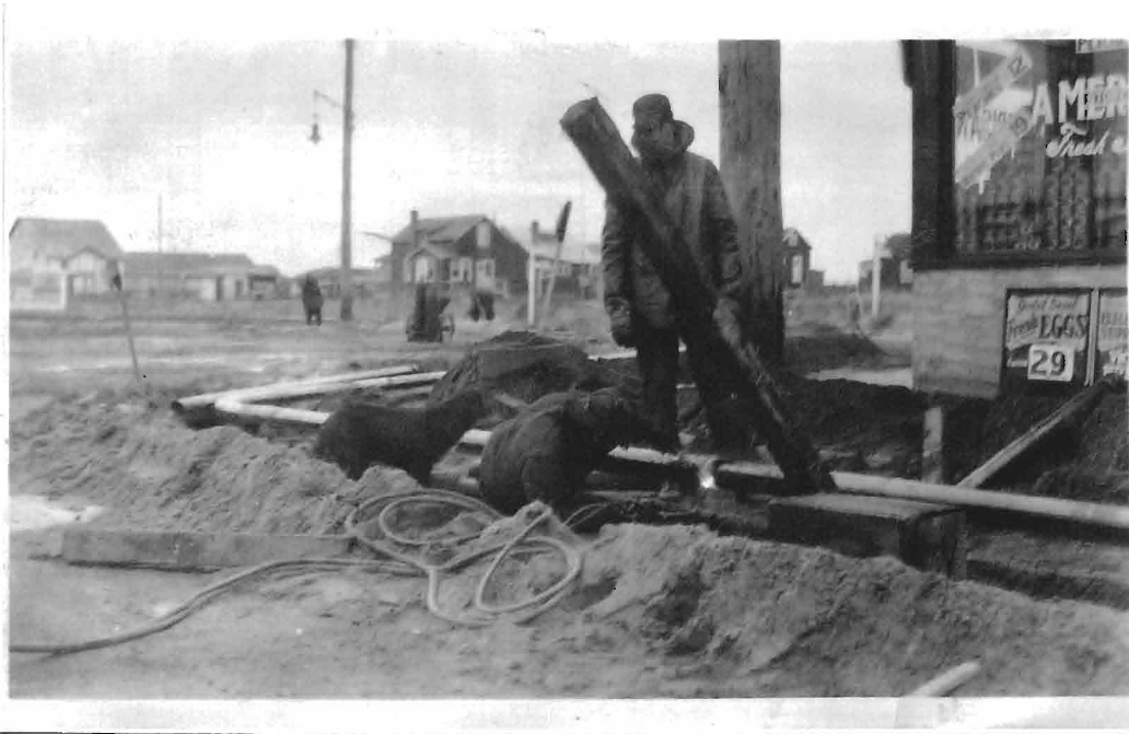
Welder Tying in 90° Bend with Overhead Weld on 4" Butane Gas Line
