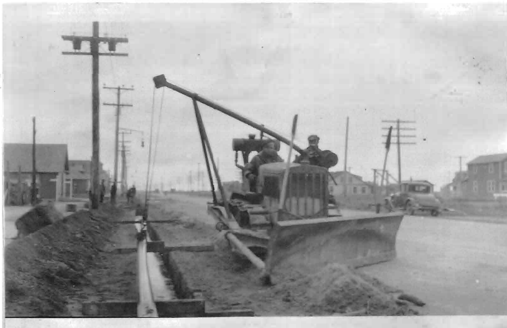
Bulldozer and Boom Equipped Tractor Lowering Pipe at Beachaven, New Jersey
