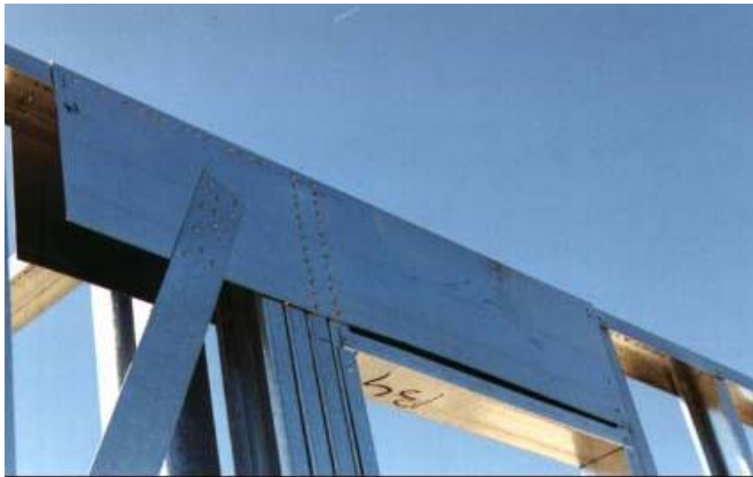
Figure 1 – Typical Steel L-Header
