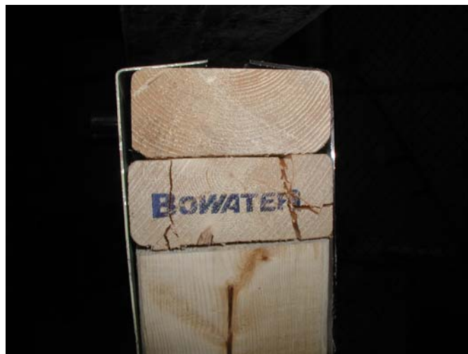
Figure 9 – Top Plate at Ultimate Load
