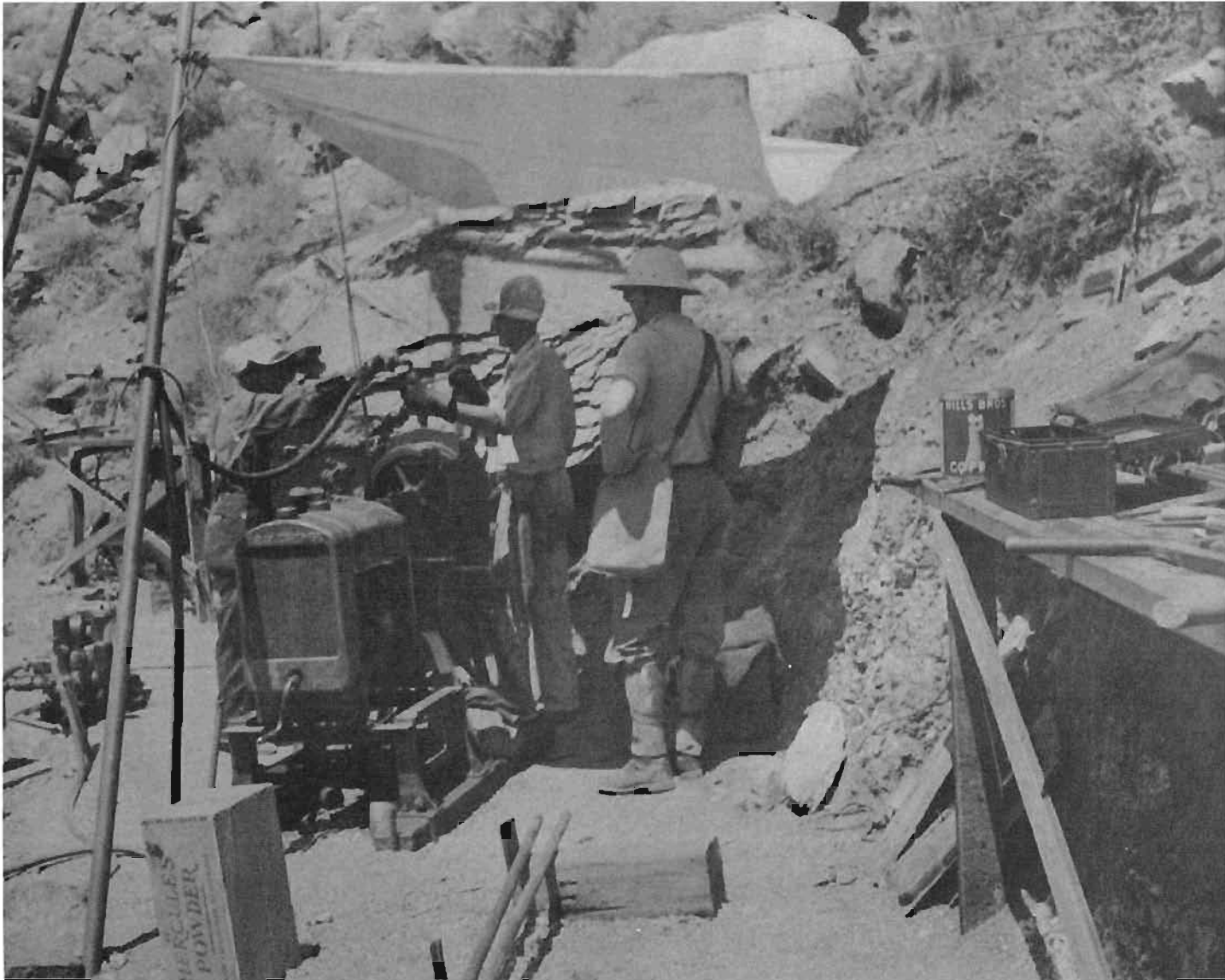
Figure 1.- Diamond drilling at Great Eastern claims.
