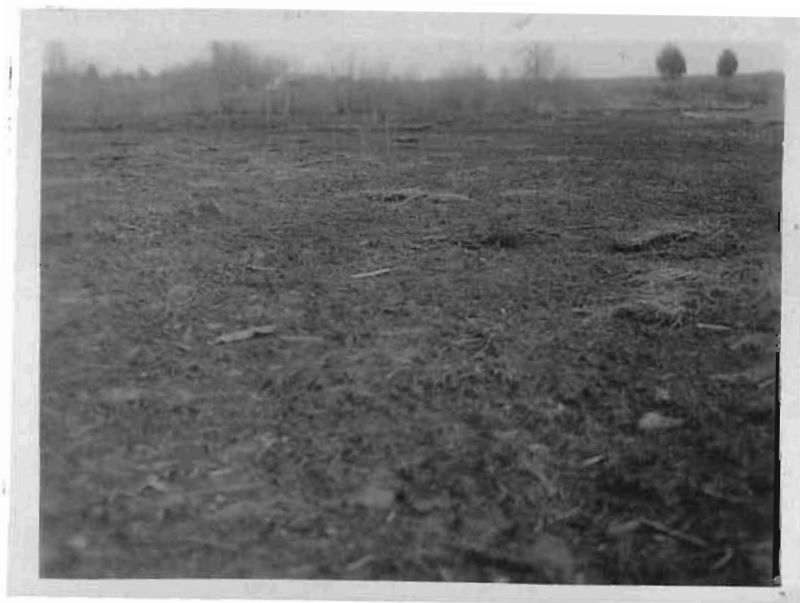
Shoreline condition after conditioning with team drawn mowers. This area is ready for wind-rowing and burning.
