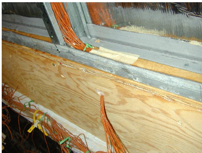
Figure 18 – Typical Split Track (Angles)
