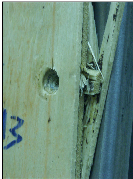
Figure 2.17: Wood Bearing Failure in Test Wall 39C
