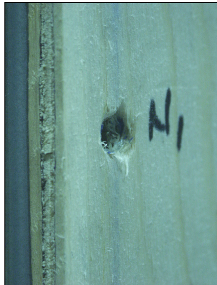
Figure 2.6: Over-driven Sheathing Screw in Test Wall 40C
