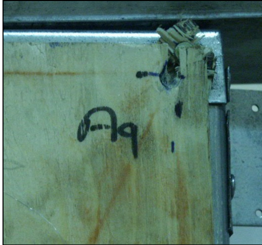
Figure 2.18: Tear-out of Sheathing Failure in Test Wall 35E
