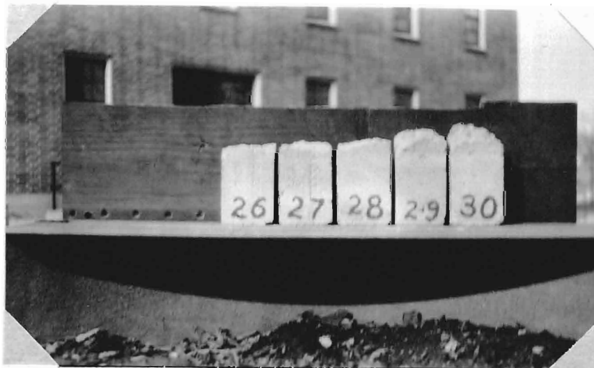
Figure 4 Laclede King Brick after subjection to the A.S.T.M. Spall Test.
