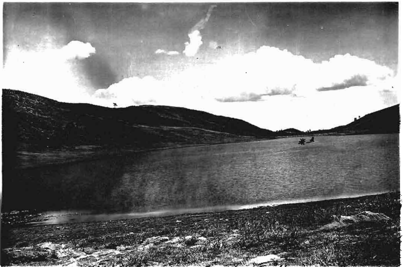
* North Lake Dam - Looking South
