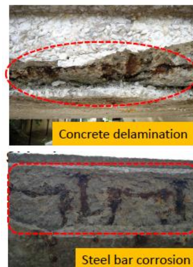
Steel bar corrosion
