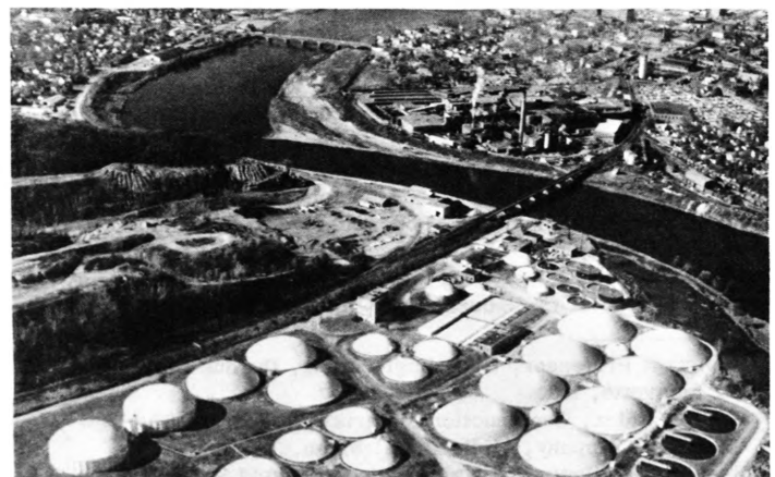
Fig. 5. 27 Spiral Generation Domes - Sewage Treatment Plant, Cedar Rapids, Iowa
