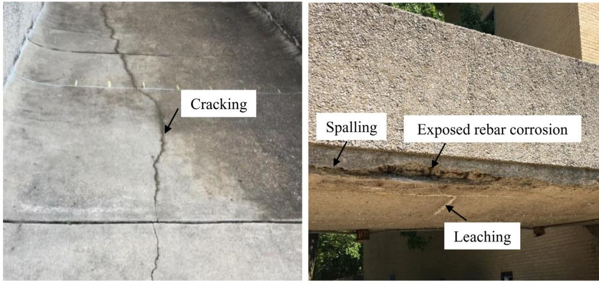
Figure 1: Bridge deck deterioration
