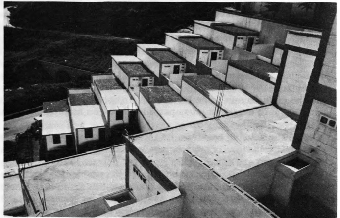
Fig. 4. Completed Group of Housing Units
