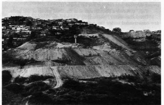
Fig. 2. Construction of the Berms
