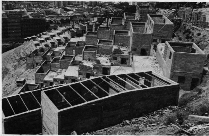
Fig. 3. Construction of the Housing Unit
