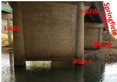
Figure 6 The I-44W Roubidoux Creek Bridge
