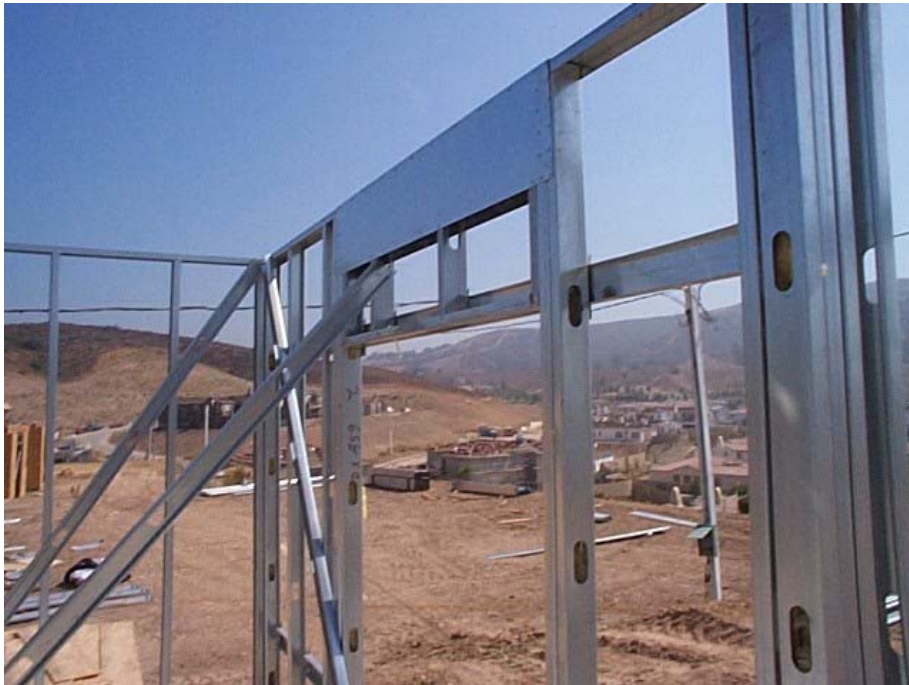
Figure 1 – Typical Steel L-Header
