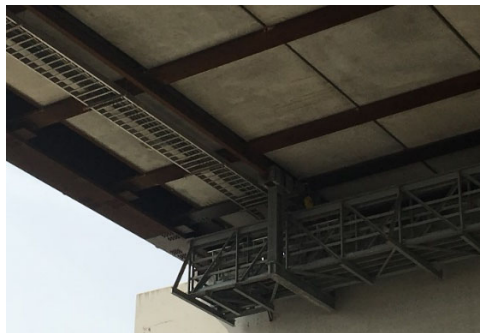
(a) Inspection platform used in practice
