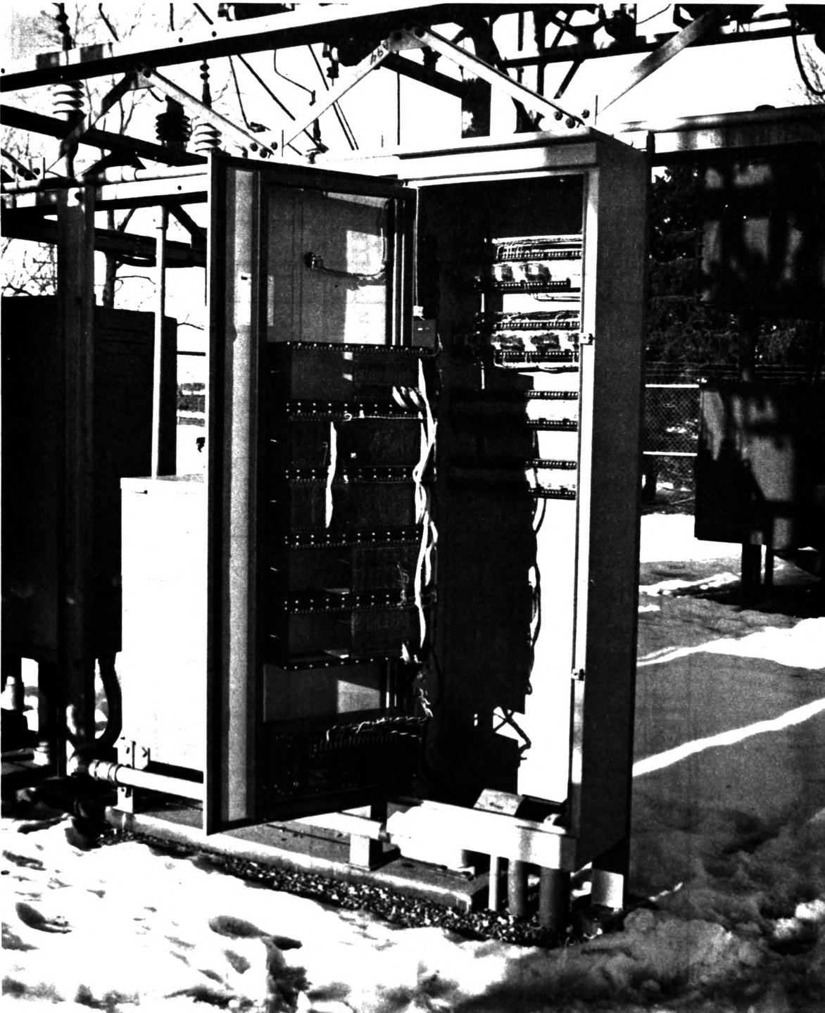
REMOTE TERMINAL UNIT - INSIDE VIEW (NOTE ROOM FOR FUTURE EXPANSION)
