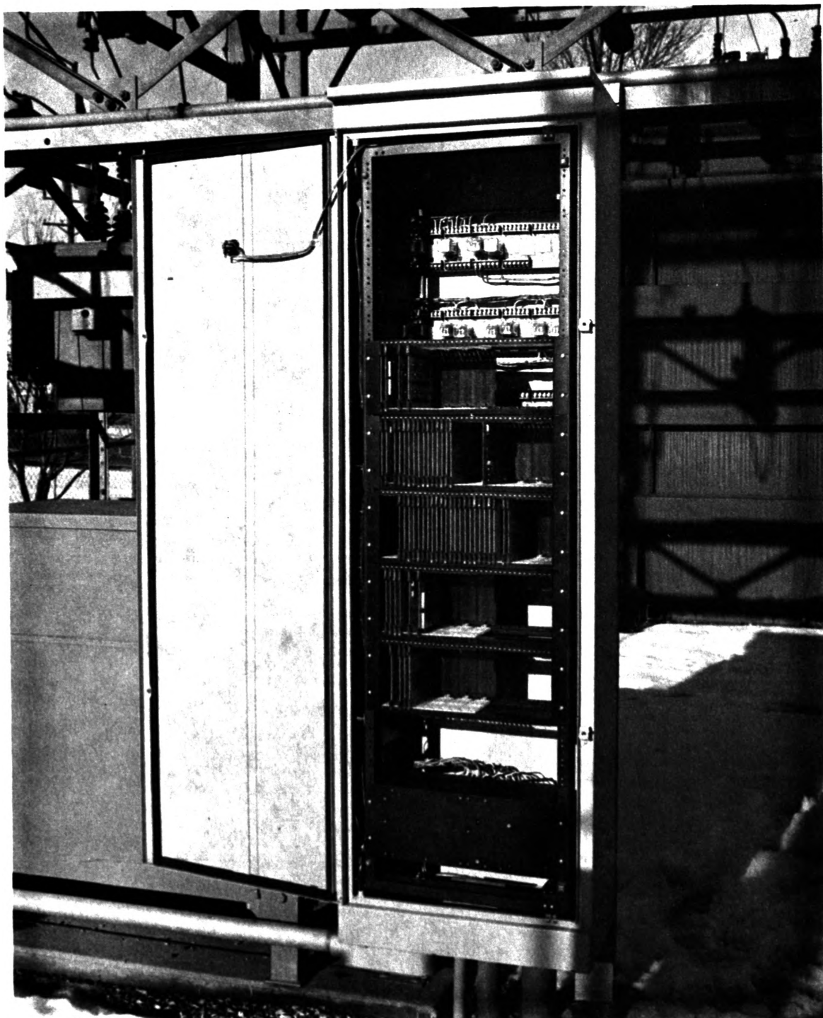
REMOTE TERMINAL - FRONT VIEW (NOTE ROOM FOR FUTURE EXPANSION)
