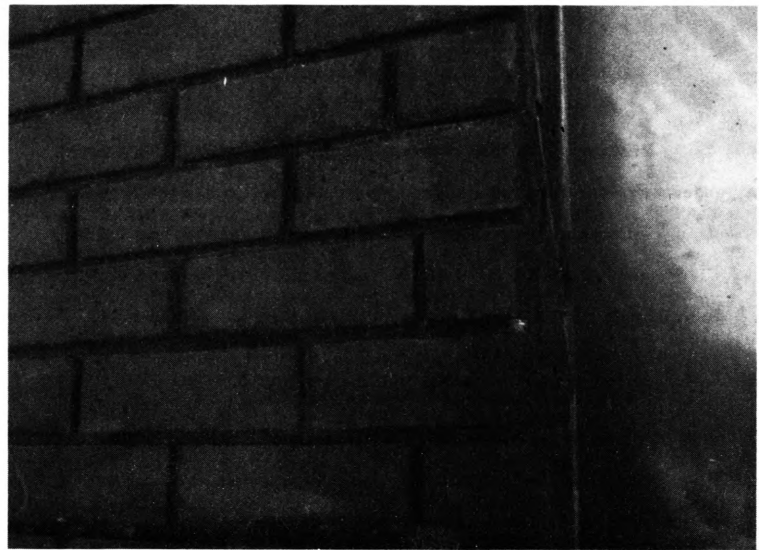
TYPICAL SURFACE TREATMENT AS CAST ON OUTER SURFACE OF A WALL PANEL
