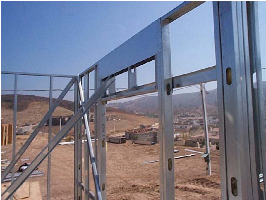
Figure 1 – Typical Steel L-Header
