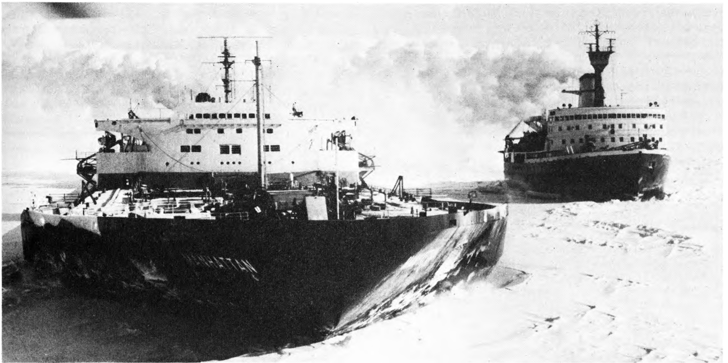
Figure 2. DOUBLE CRUNCH -Humble Oil & Refining Co.'s icebreaking tanker, the SS Manhattan, and the Canadian Ministry of Transport's newest icebreaker, the Louis S. St. Laurent, crunch through the snow-covered ice of northern Baffin Bay. The Manhattan is completing its second Arctic voyage to collect data for use in determining the economic feasibility of transporting Alaskan crude oil through the ice-covered Northwest Passage to the U.S. East Coast.
