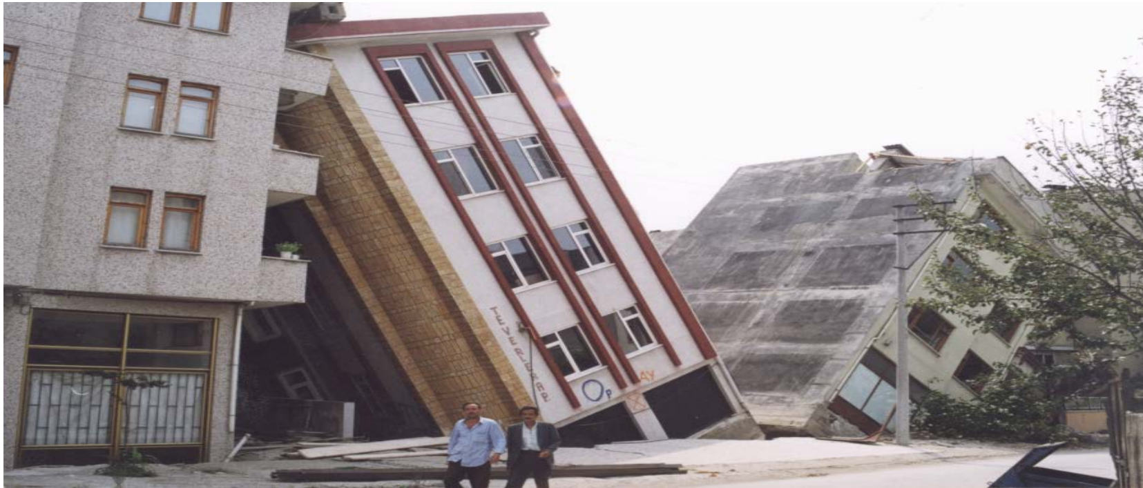
Examples of bearing capacity failures of shallow foundations in Adapazari (Yilmaz et. al. 2004)
