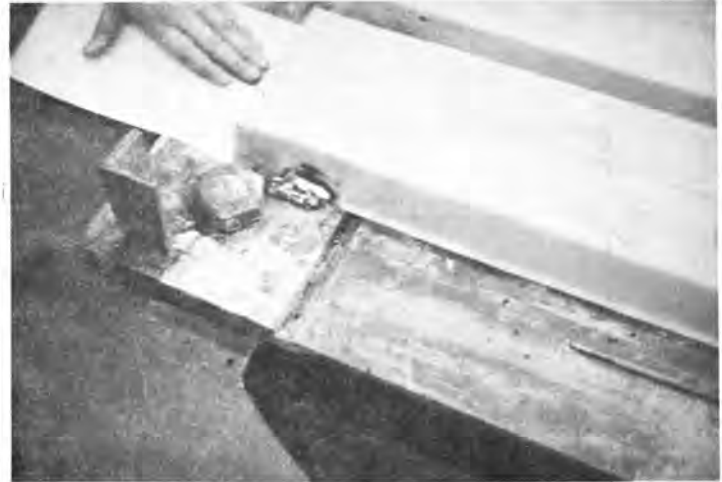
Fig. 9. Tearing of Sheet Around Weld and Displacement
